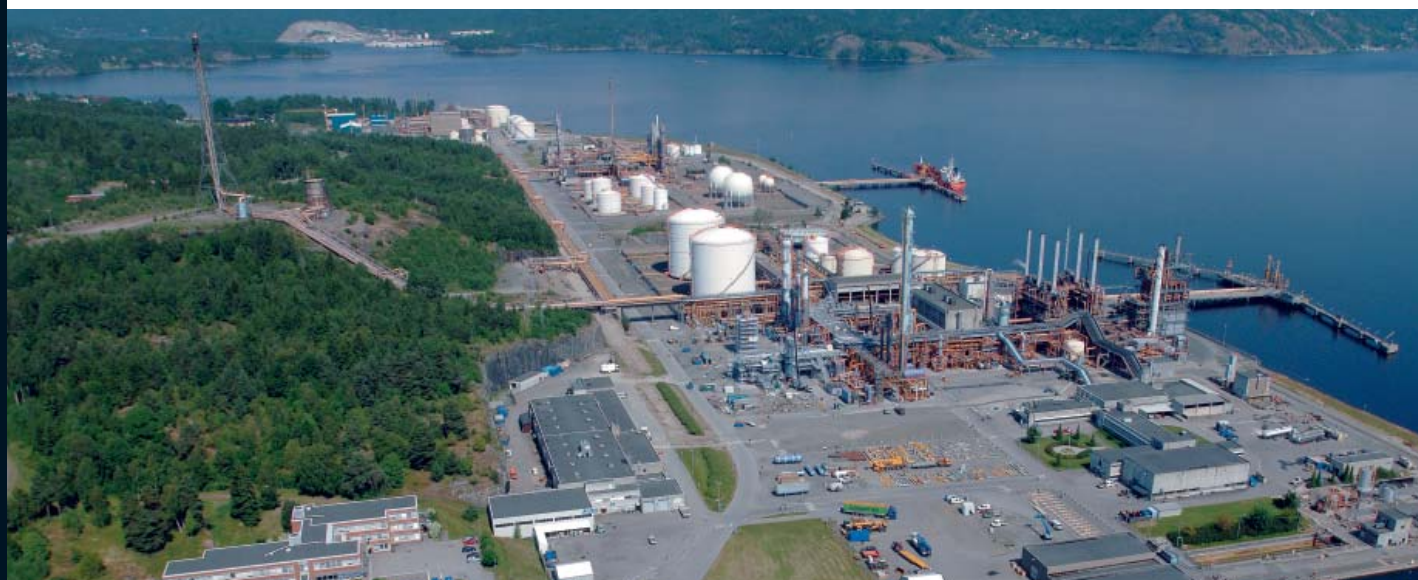
Hydro Polymers Rafnes Industrial site
